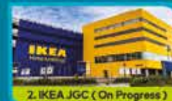
2. IKEA JGC ( On Progress )
